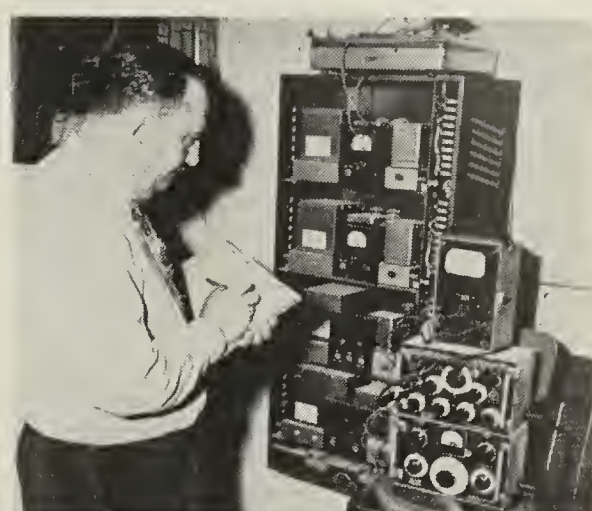
The Altec service man makes a complete transmission test while on the job in the Melroy's booth.
